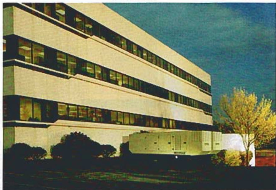
An effective UPS system should have at least one generator behind it to make sure the system operates and functions properly 24/7.
